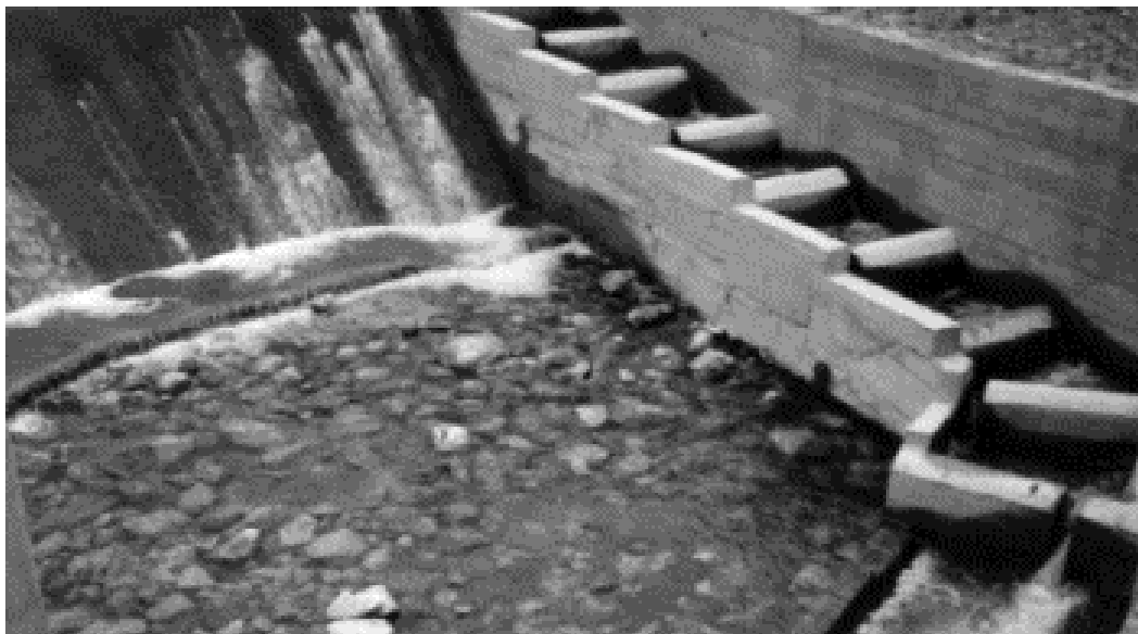
Photo 7.14: Fishpass with vertical slots
