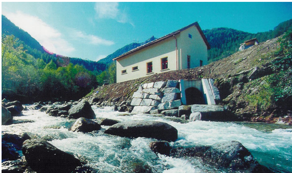
Photo 6.1: Overview of a typical powerhouse
