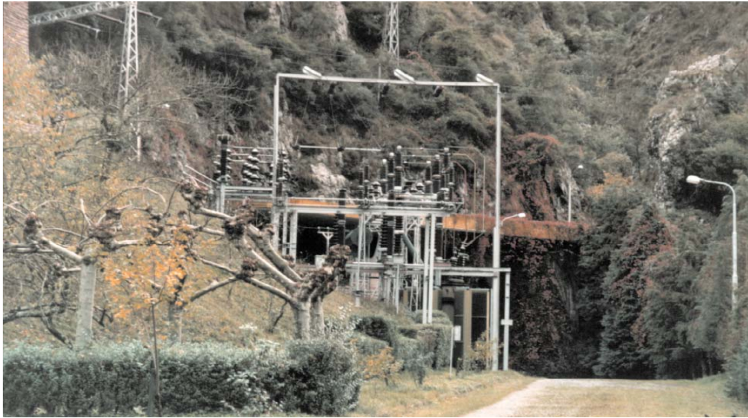
Photo 7.18 Visual impact of outdoors substation
