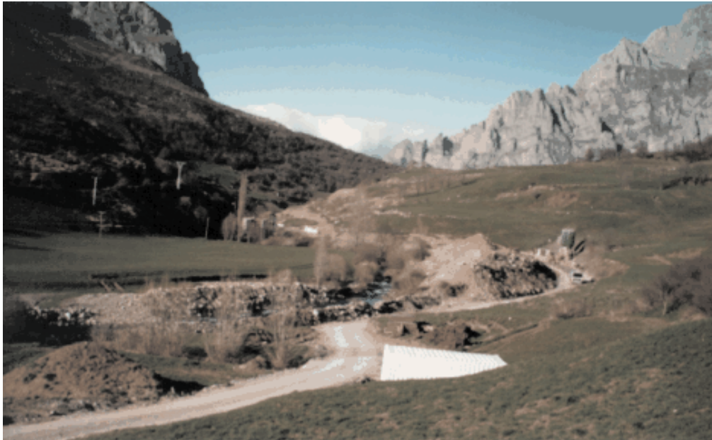
Photo 7.5: Construction phase – excavation
