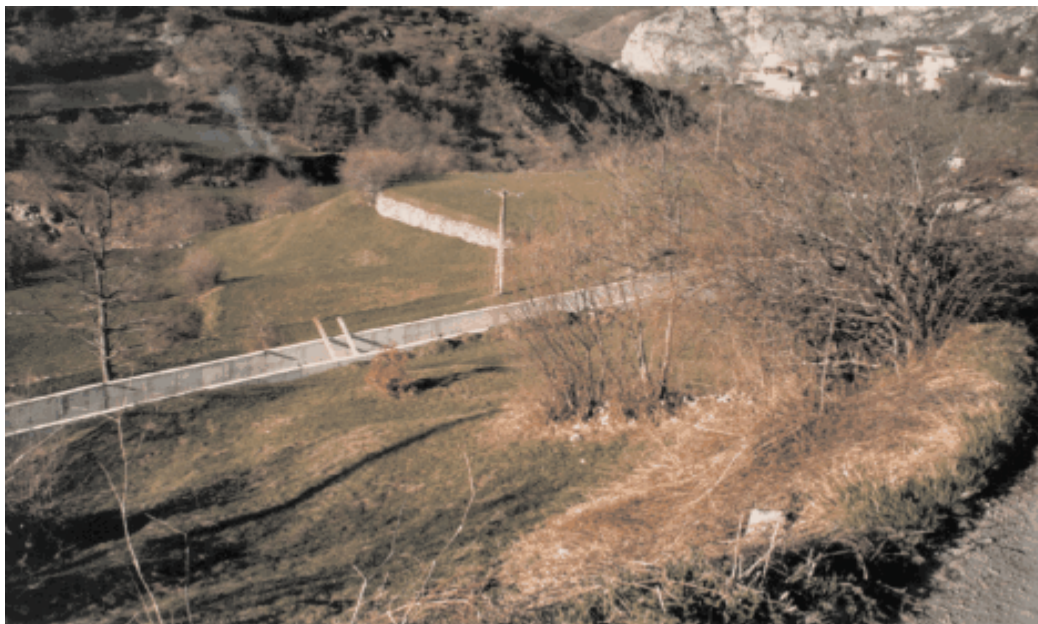
Photo 7.6: Construction phase – concrete canal
