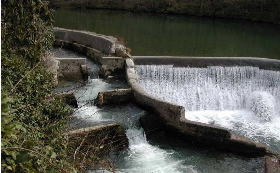
Photo 7.13: Fishpass of rustic construction
