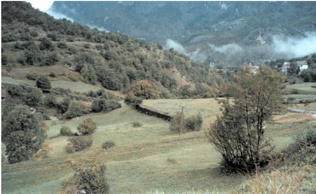
Photo 7.7: Construction phase – canal complete
