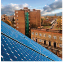
Community owned solar panels in Brixton, London.
